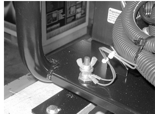
Figure 3-1. Grounding the Generator
